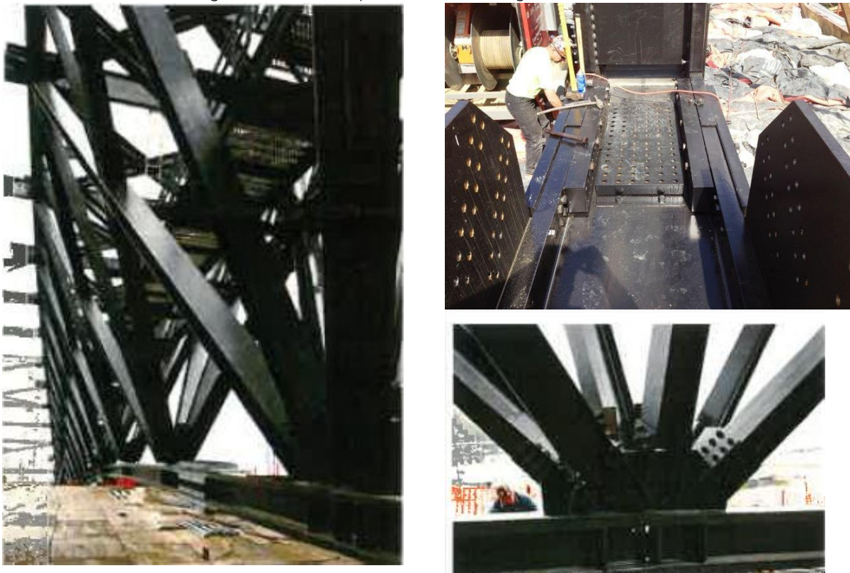
Figure 3-20. Example of jumbo sections used in trusses connections: a) New Pacific NW Pacific Ballpark; b) Chase Field (Formerly Bank One Ballpark) in Phoenix, AZ. Fabricator: Schuff.
