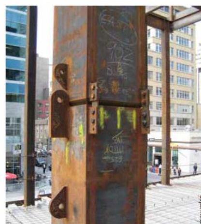
Figure 3-4. Splice connections – interrupted zone [33].
