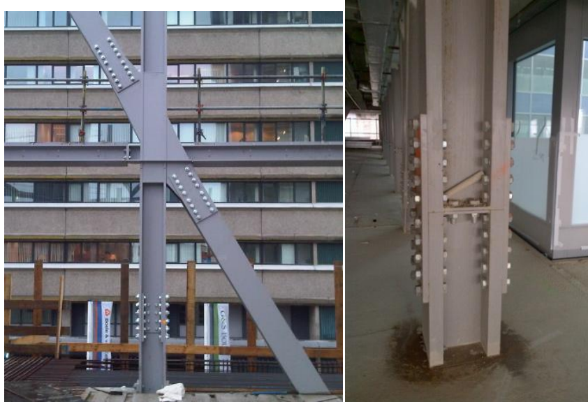
Figure 3-12. Connections submitted to compression loads – STADSKANTOOR – UTRECHT.
