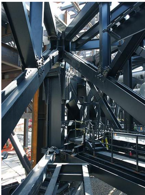
Figure 3-21. Example of jumbo sections used in trusses connections: Chase Field (Formerly Bank One Ballpark) in Phoenix, AZ. Fabricator: Schuff.
